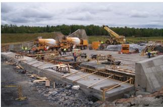
RIZZO developed a spillway redesign for the Silver Lake Reservoir Dam. The new spillway design balanced various constraints including environmental impact, hydro power output, construction cost,
